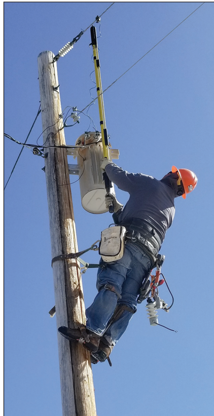
Foreman Jim Richter energizes a transformer.
