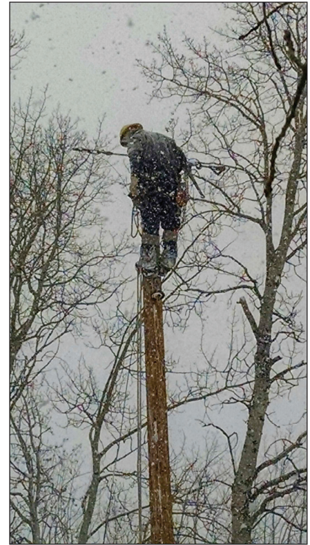
Lineman Tyson Ruff repairs a power line during a storm.
