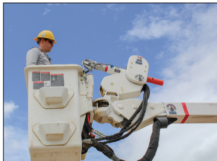
Casey Kombol works bucket controls.
