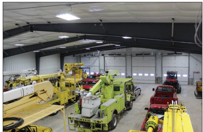
FEC trucks and equipment are neatly parked inside the new, heated truck garage.
