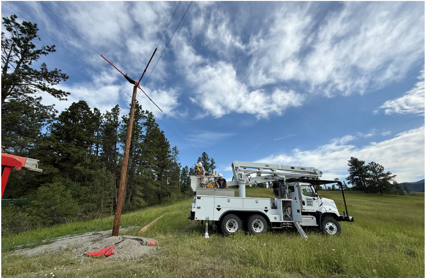
Fergus Electric lineworkers Darek Dygert and Travis Sura work in the Ruby Gulch area. | PHOTO BY MARK SCHWOMEYER
