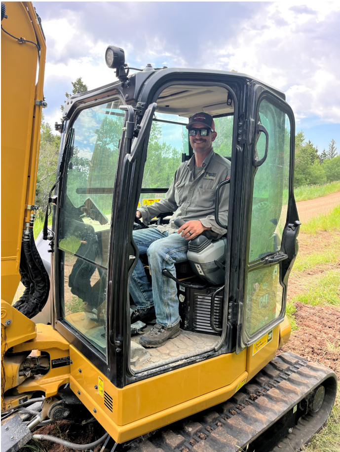
Foreman Owen Thatcher digs in an underground powerline up Swimming Woman Road. | PHOTO BY DYLAN RICKMAN
