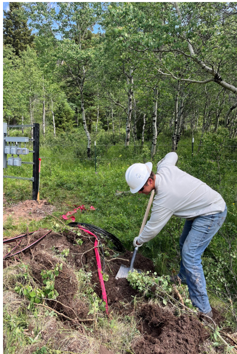
Dylan Rickman works on an underground powerline job up Swimming Woman Road | PHOTO BY OWEN THATCHER
