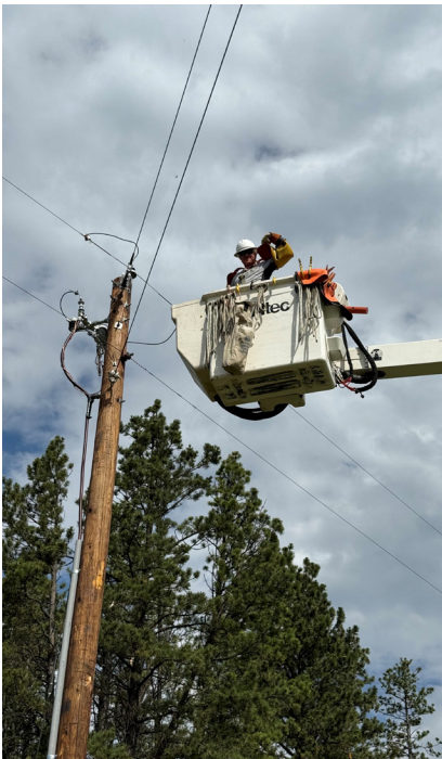
Lineman Darek Dygert works on a powerline in the Ruby Gulch area. | PHOTO BY MARK SCHWOMEYER
