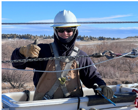
Journeyman Lineman Dan Rice. | FERGUS ELECTRIC PHOTO
