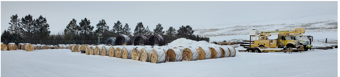
Fergus Electric is accumulating material for upcoming underground cable replacements. | FERGUS ELECTRIC PHOTO
