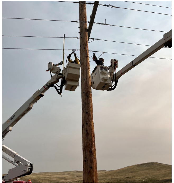
BELOW: Transformer Repairman Mark Schwomeyer, left, and Lineman Darek Dyger install a conductor on new powerline.
