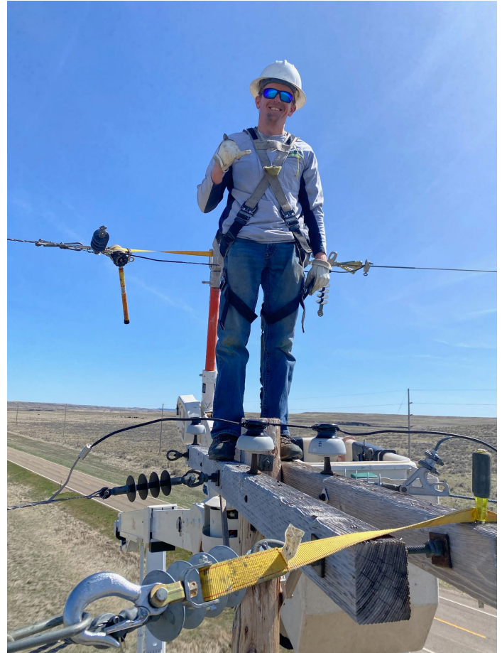
Journeyman Lineman Dakota Wahl is getting ready to deadend wires during a pole replacement procedure.
