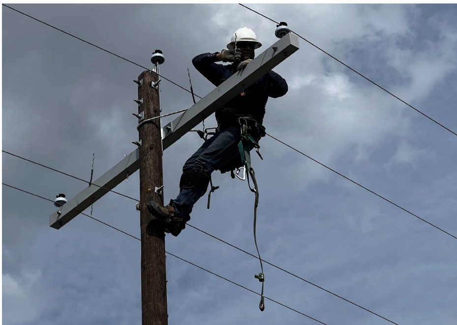
Apprentice Lineman Jason Deffinbaugh is tying a phase on a new three-phase line. A number of infrastructure projects are planned for 2026.
