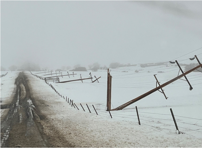
Transmission poles in the Spion Kop area were snapped all the way down the line. | FERGUS ELECTRIC PHOTO
