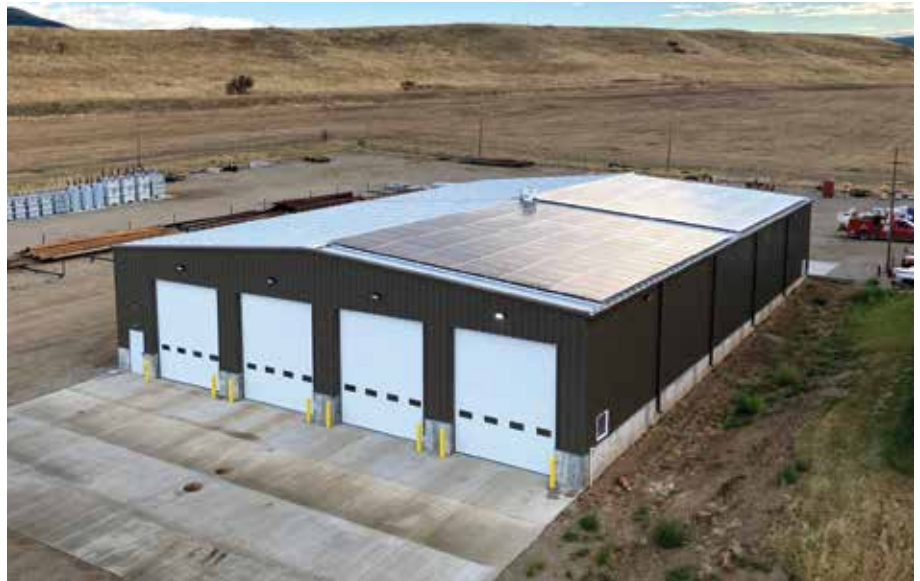
OnSite Energy completed construction on the 72kw Phase 2 roof-mounted solar array on Fergus Electric Cooperative's truck garage roof. | PHOTO COURTESY OF FERGUS ELECTRIC
